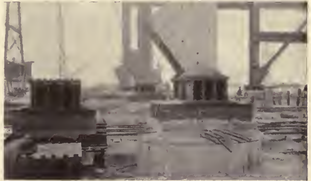
CLOSE-UP OF COLUMN FOOTINGS Showing reinforcing steel at floor beam level
